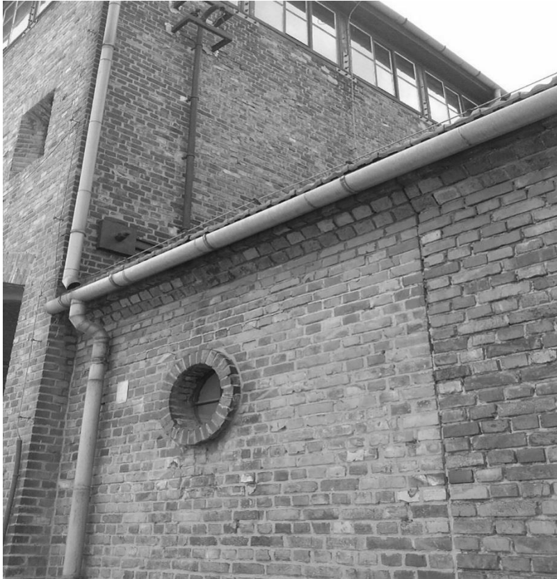
Figure 2. Zentralbauleitung, entrance, Auschwitz-Birkenau (detail of seam), c. 1943 (author's photo)
